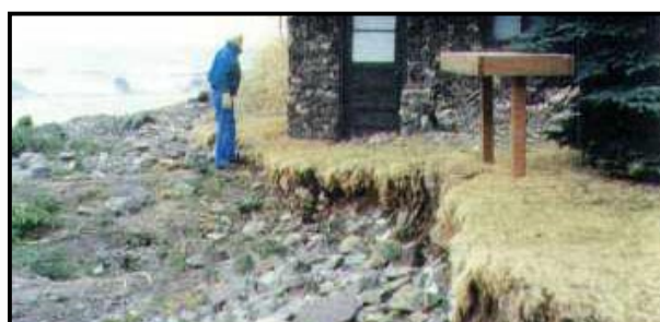
Pinned Rock Wall Method -- Before.
