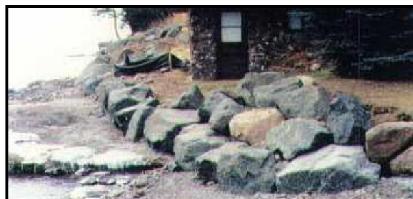
Pinned Rock Wall Method -- After. (Photos courtesy MN Board of Water and Soil Resources)
