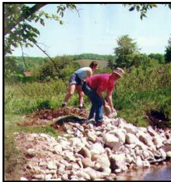
Volunteers work at an eroded site.
